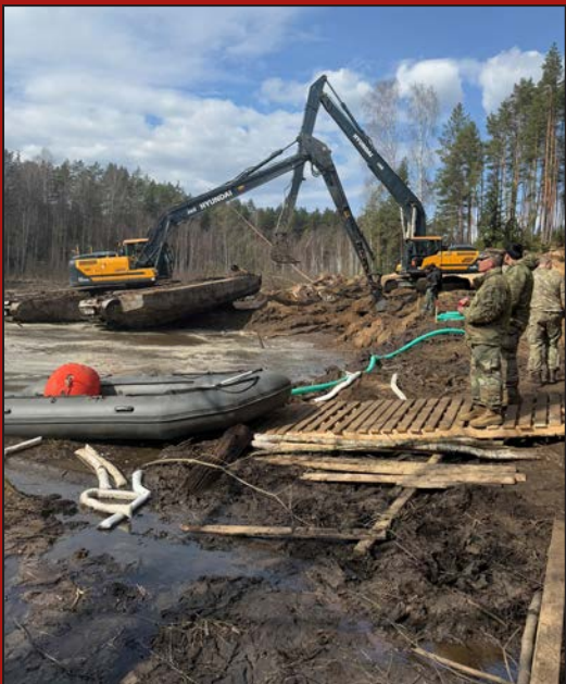
Floating excavator and land based excavator working together. Each scoop was sprayed down with water to break up and inspect, then taken away by the land based excavator.
