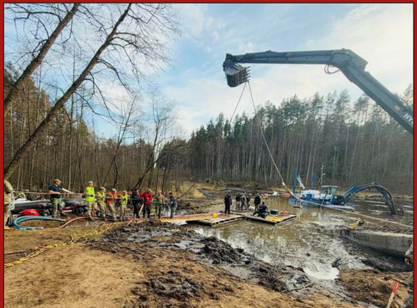
Multiple Lithuanian Engineers and US Divers work together to place lifting slings near dive location.
